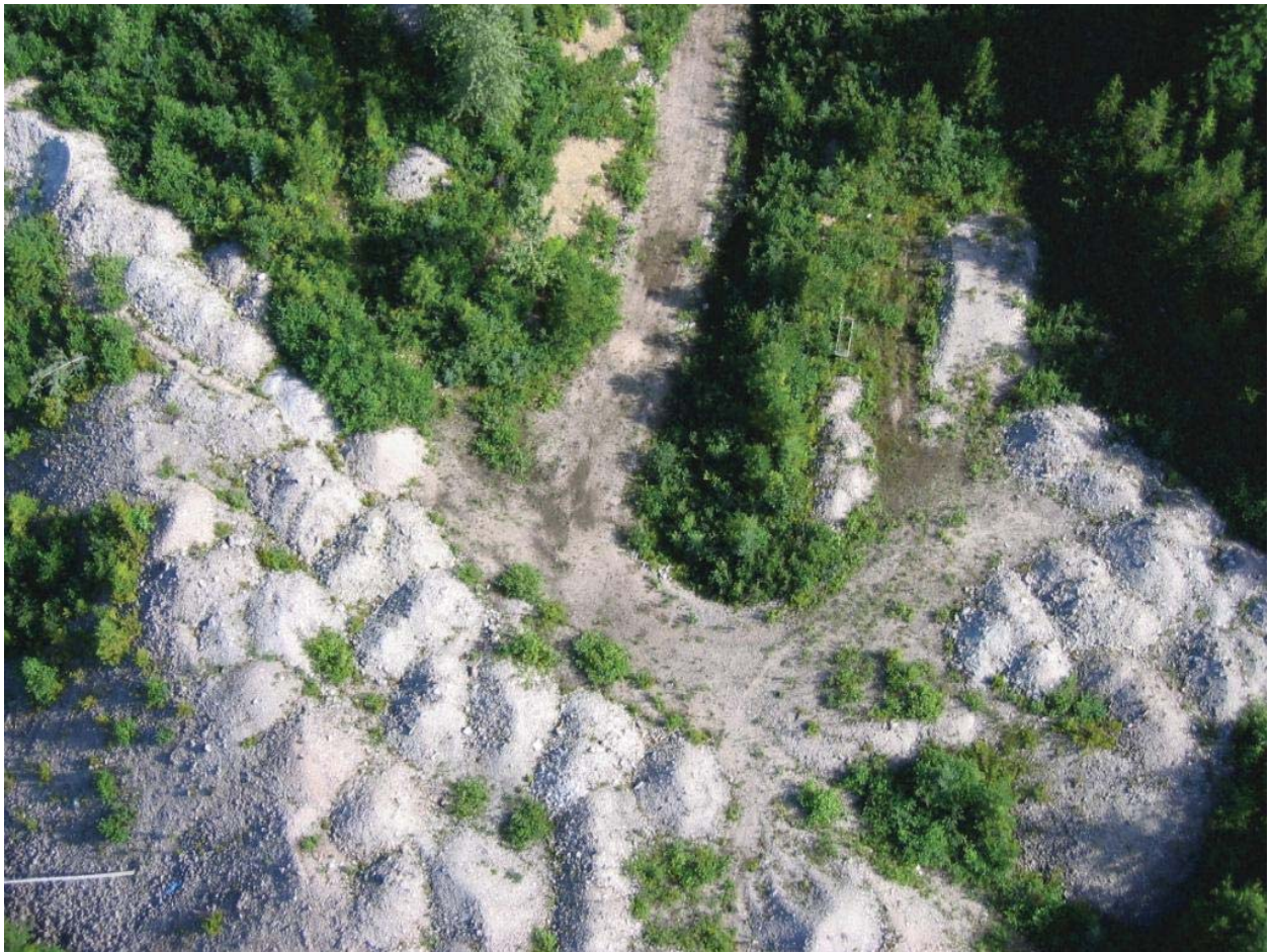
Adit 2 muck piles
