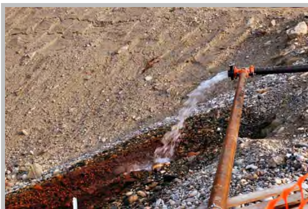
Figure 1. Water discharge into settling pond, with iron staining on cobbles. The pipe is 4". Figure 2. Pile of clean cobbles to supply rock for the discharge apron.
