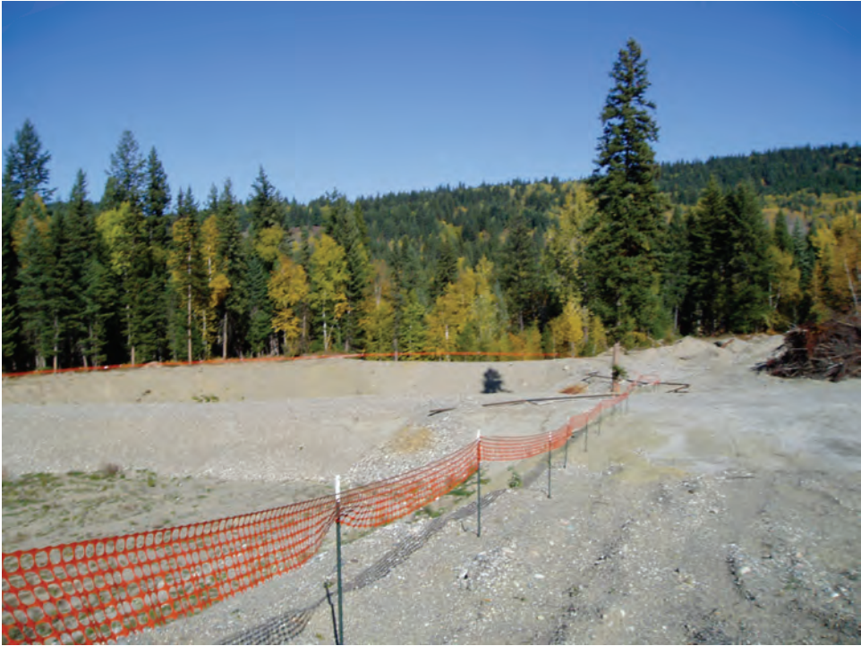
Top Left: Safety fenced rehabilitated settling (near left and ex-filtration) pond
