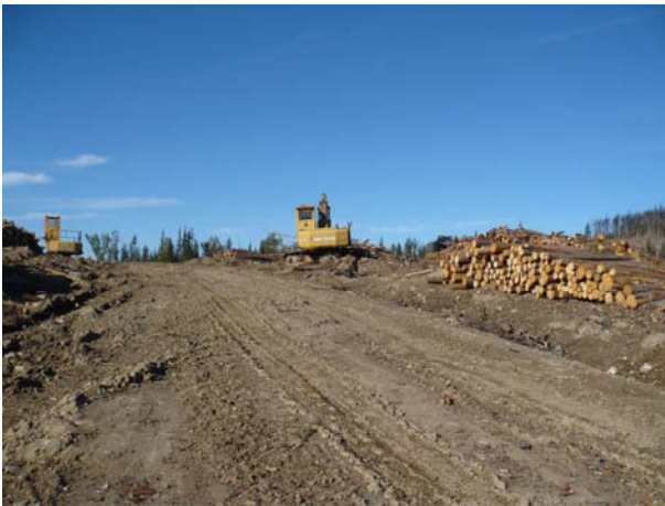
Station 7 : Current logging operations – new northern access opened
