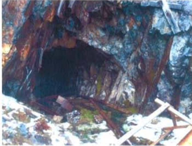
Photo 11: Portal before debris removal and culvert installation
