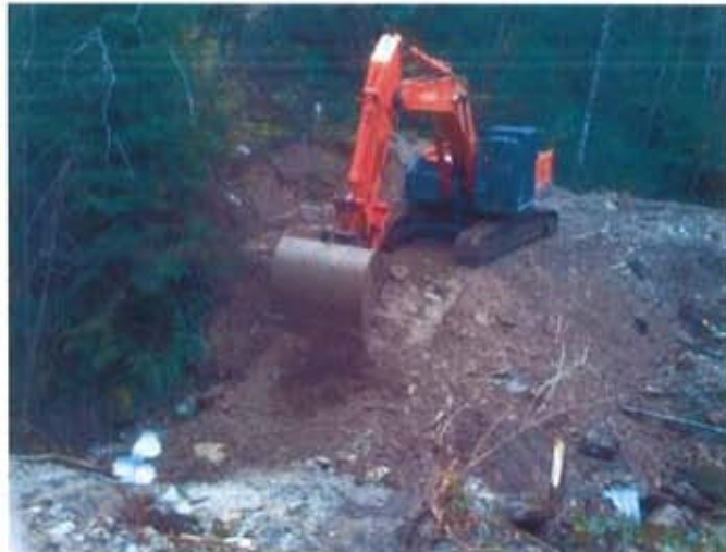
Photo 3: Installation of 2x1000 CMP on creek 25
