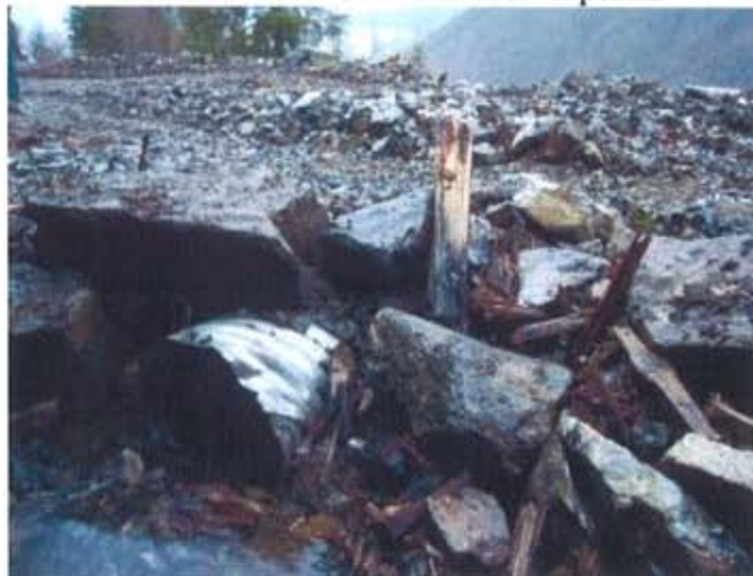
Photo 12: 600 CMP installed at portal
