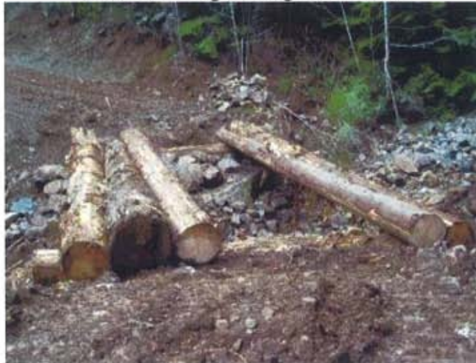
Photo 5: Bridge during construction
