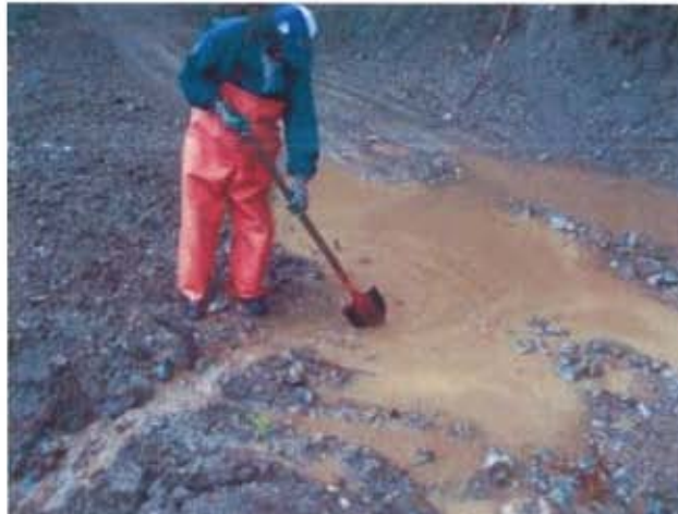
Photo 15: Road maintenance – water removal
