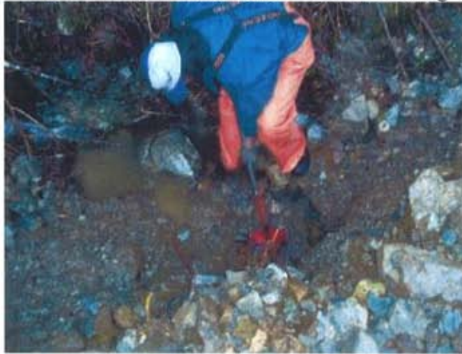
Photo 14: Road maintenance – culvert cleaning
