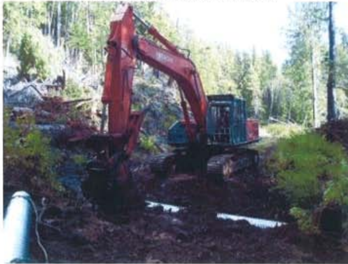
Photo 2: Culvert Installation
