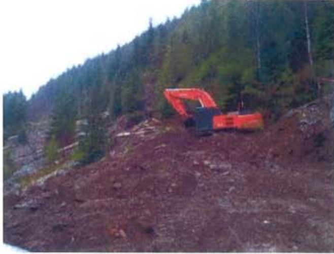
Photo 10: Reactivation of resloped road just before portal
