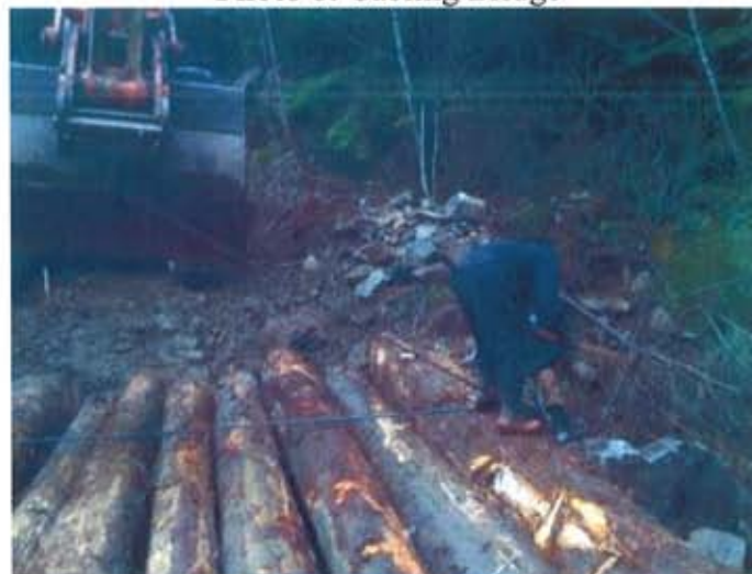
Photo 6: Cabling Bridge
