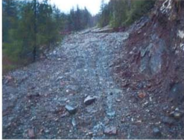
Photo 13: End of road reactivation and turnaround
