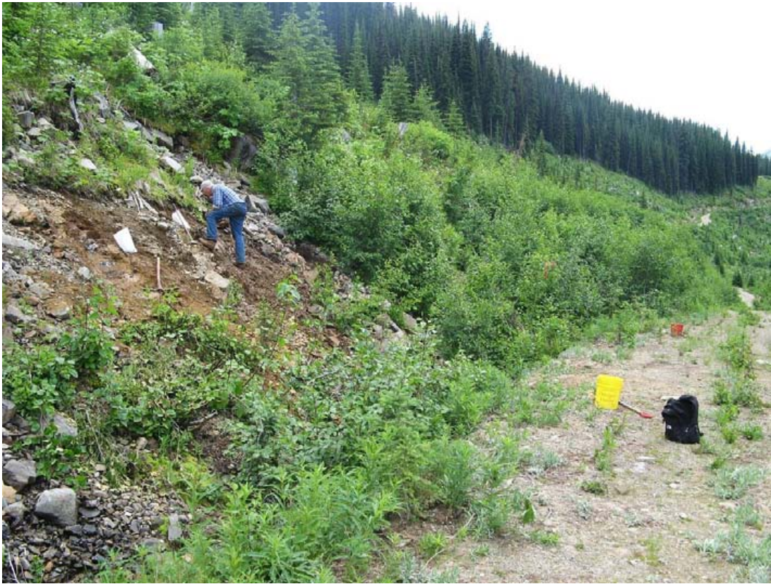
Plate 8 View South. Site of SVE2 & SVE3. 21km Hidden Creek FSR. Grant Crookes.
