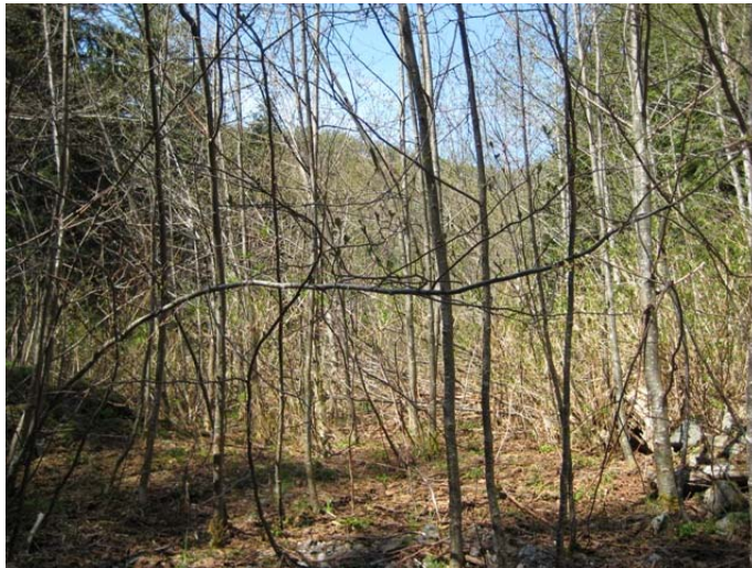
Picture 6: Beano Overgrown Road
