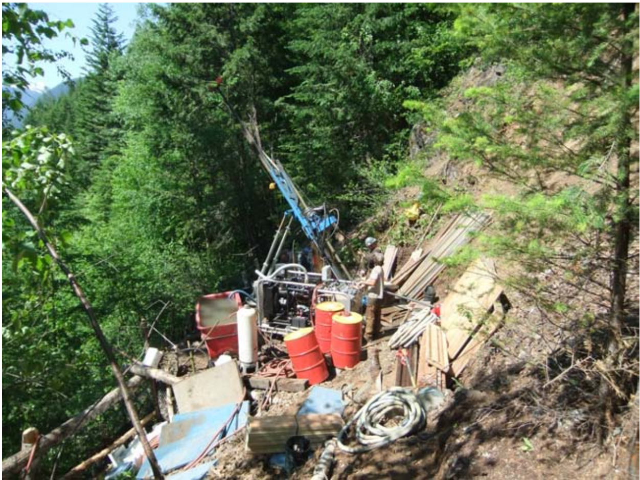
Photo 5: Drilling from drill pad 1 testing the DOT Zone.
