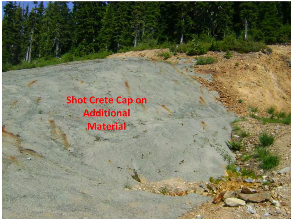
Fig 7 – Bulk Sample covered by shotcrete
