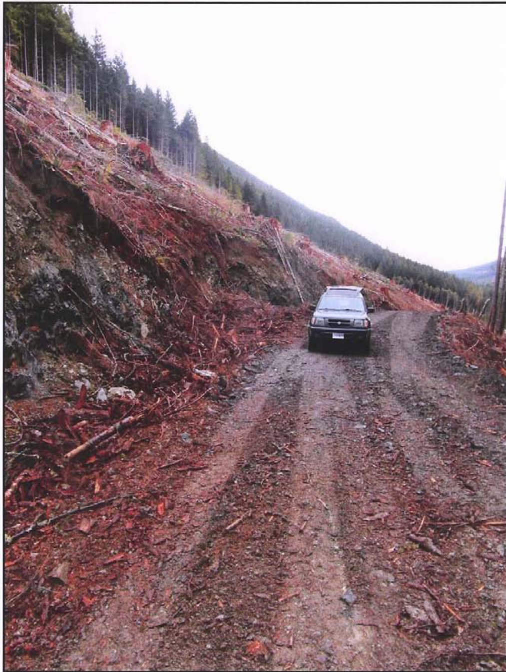
Photo 8: Newly exposed bedrock in Forestry Spur road within new cut block. Vicinity of Sample # 111069
