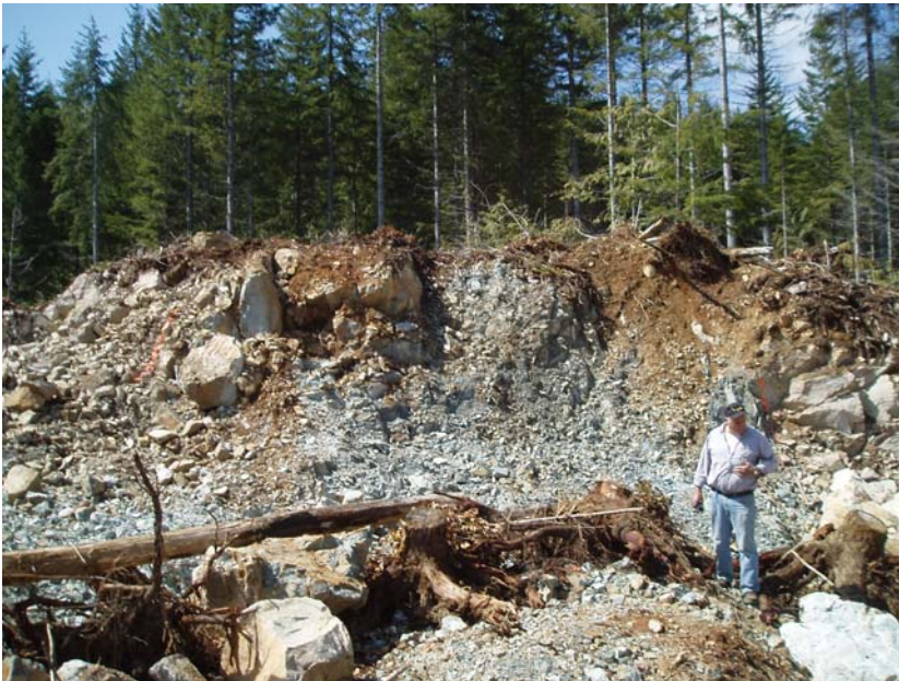
Photo 1: Showing #4 at north end of Line G7
