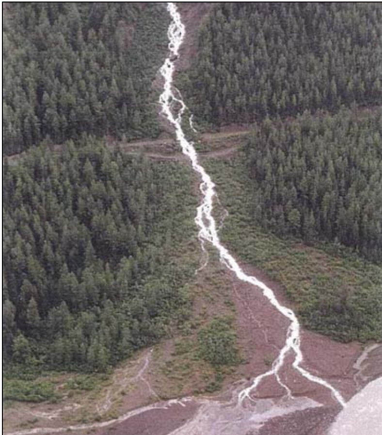
Figure 18-2 Road Crossing of Hartley Gulch Creek
