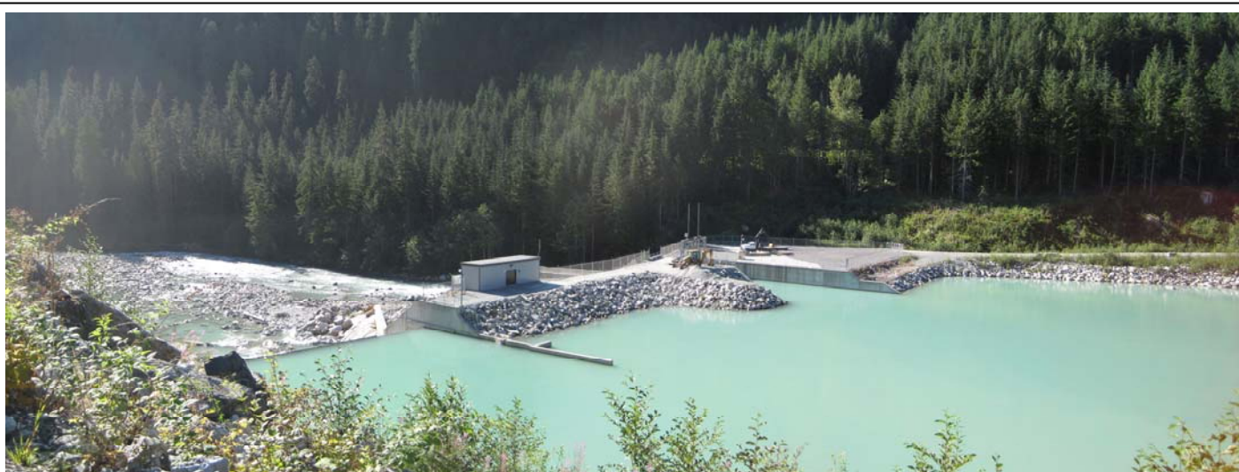
Photo 2: View of the run-of-river intake facility of the Ashlu Green Power Project, located just inside the east boundary of the Ashlu Property. Photo looks southeast taken from the Ashlu North road. Service vehicles near center of image serve for scale.
