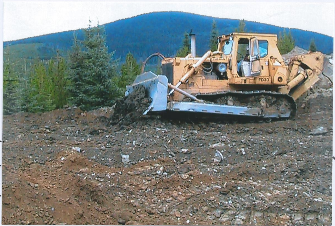
stripping off overburden #7
