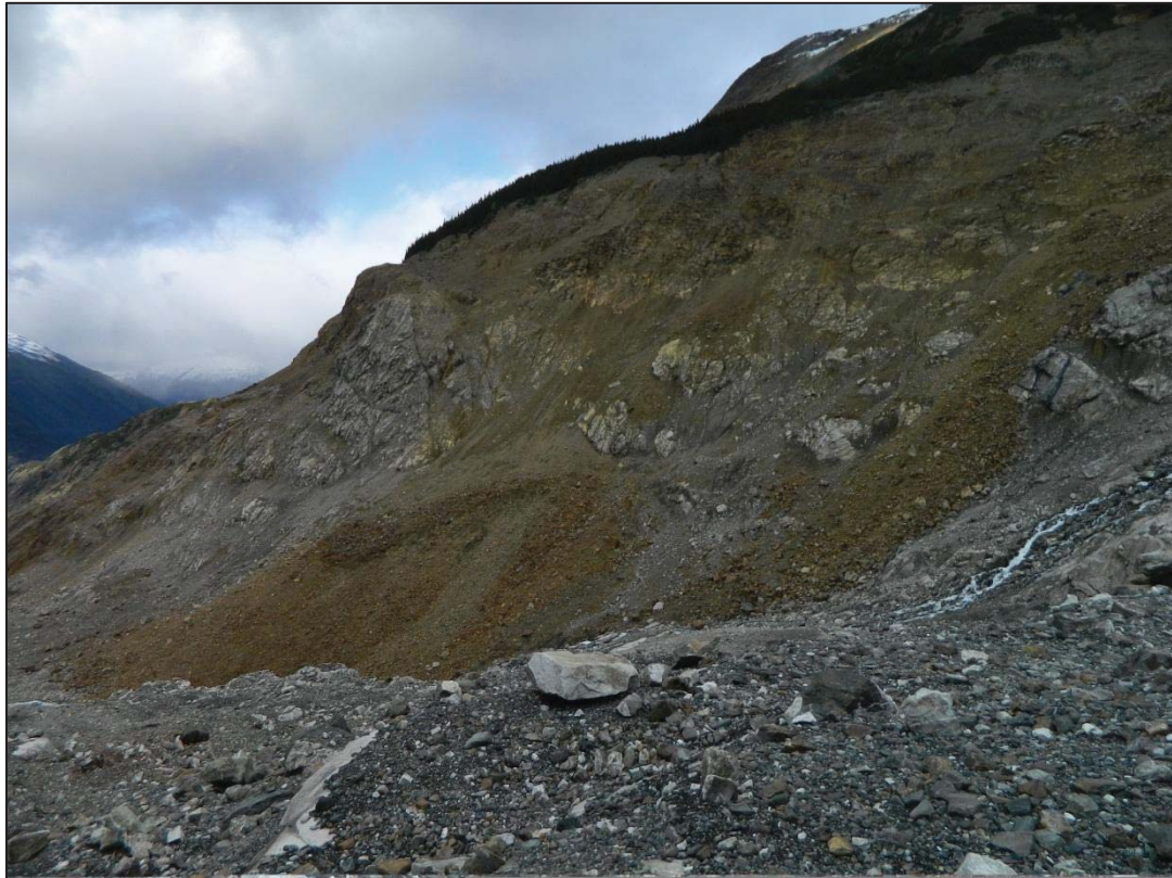
Figure 6-5 Photo of Rockfall at North Side of Lost Valley
