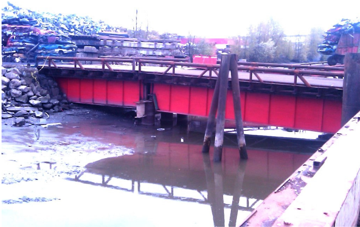
Figure 4: Example of Pitt River Bridge girder deployed in an access ramp application.
