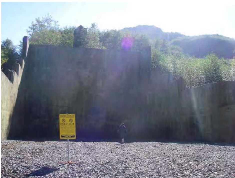
Photograph 16: Foundation walls for old concentrate storage building near proposed marine berthing location.
