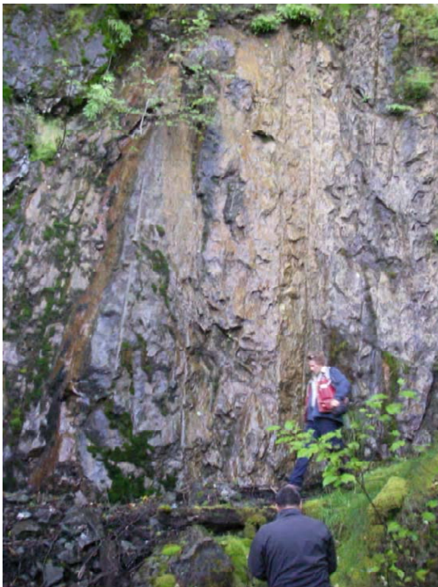
Photograph 5: Shows old bedrock face that has been blasted below Pit No. 1 on road access. Seepage over the face is forming a carbonate rich coating on the rock.
