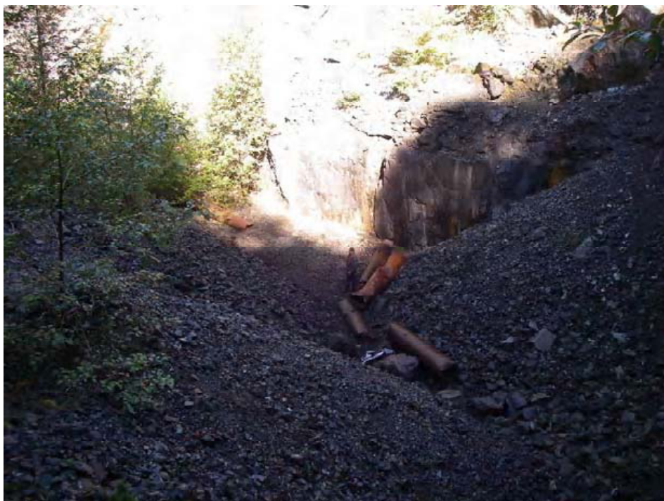
Photograph 11: View into bottom of Pit No. 1. Old underground opening is to the left of photo but has been buried under waste rock to prevent entrance into the workings.
