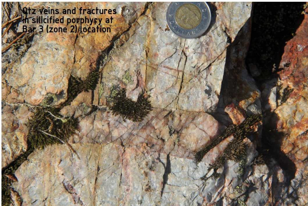
Figure 8.15: Mm to cm scale quartz veins and accompanying fractures cutting silicified rhyolite porphyry.
