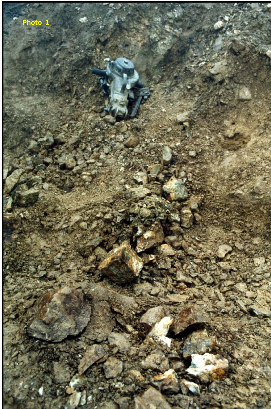
Photo 1 above shows process of re-opening old trench 'A' on the North Master Ace zone with exposed quartz-carbonate veins and malachite staining. Trench contains highly decomposed iron carbonate, talcose schist.
