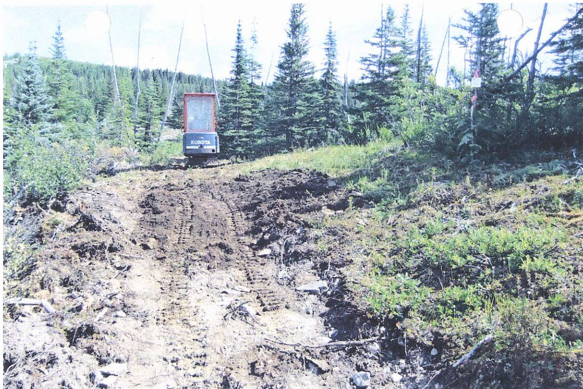
Trench # TR10/13 Filled in
