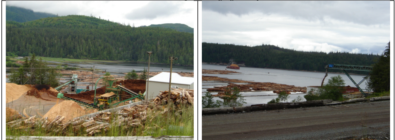
Plate 2 . Northland Power's woodchip and barging facility at Beaver Cove.
