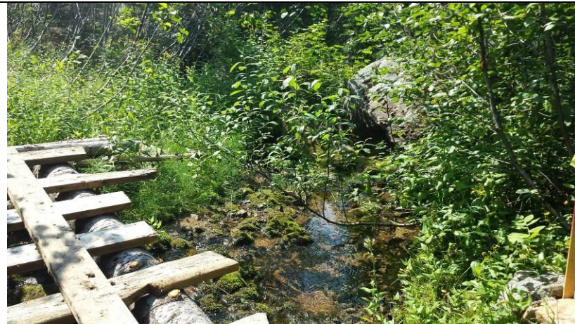
Photo 7. Temporary bridge crossing of Fingland Creek at F4.
