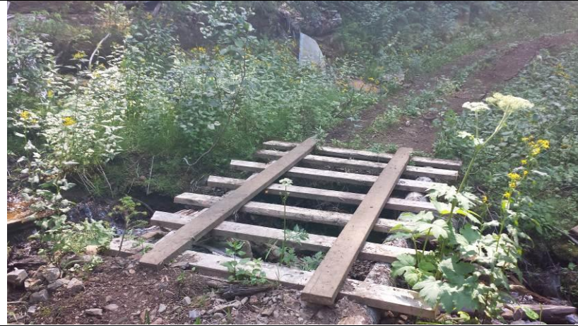
Photo 5. Temporary bridge crossing of Fingland Creek at F3.
