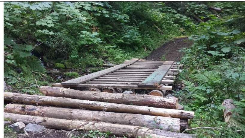
Photo 3. Temporary bridge crossing of Fingland Creek at F2.
