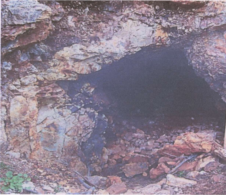
Photo 1: Photo of opening of small adit at 49^{\circ} 12' 30''\text{N} and 116^{\circ} 50' 06''\text{W} .
