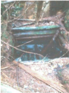
Wood cribbed vertical lift shaft – 150' depth #6
