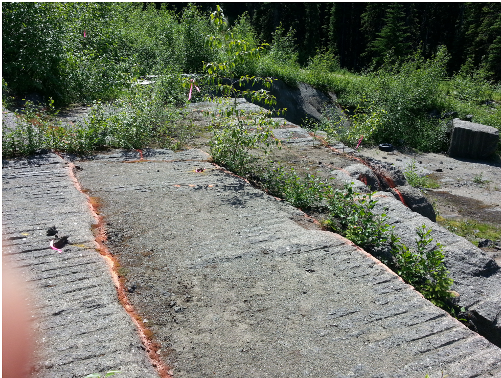
Figure 8: Line drilling between joint set 2.
