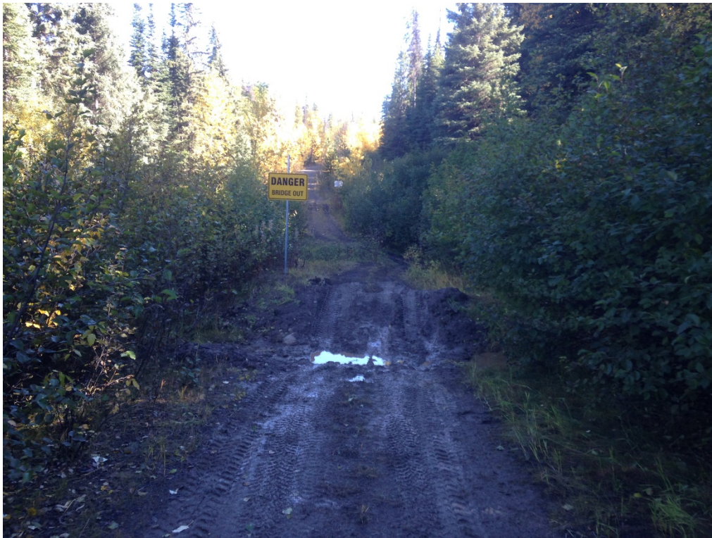
Photo 2 - One of four "tank-trap" style road deactivations on Hanson road.
