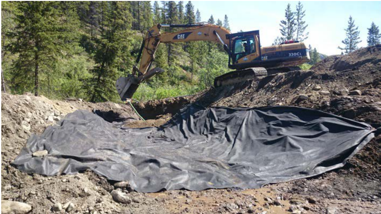
Figure 1. Excavating the stream bed for emplacement of culvert at km 22.4.
