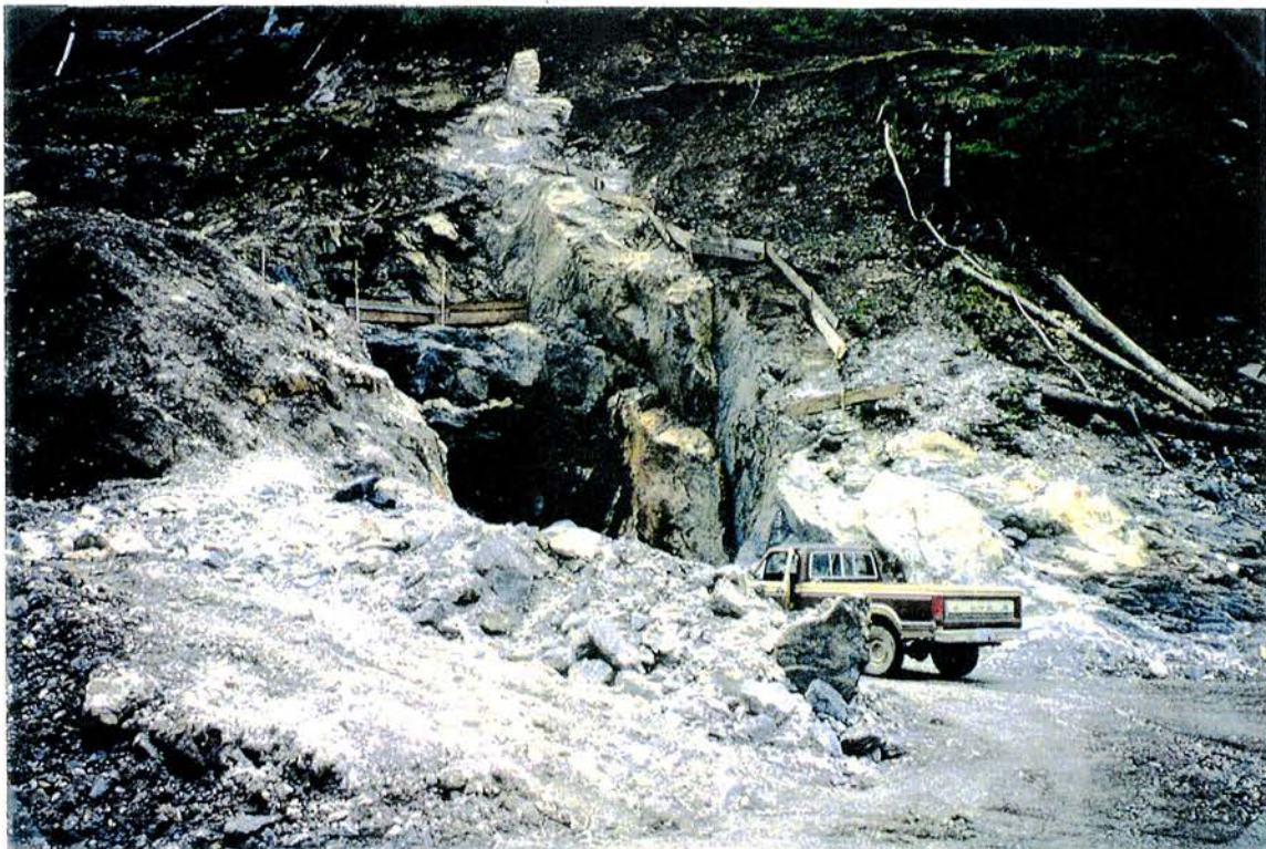
PIT AND MAIN VEIN STRUCTURE AFTER BULK SAMPLE "155 VEIN" REMAINS INTACT GRADE 11 GPT ACROSS 1 METRE WIDTH
