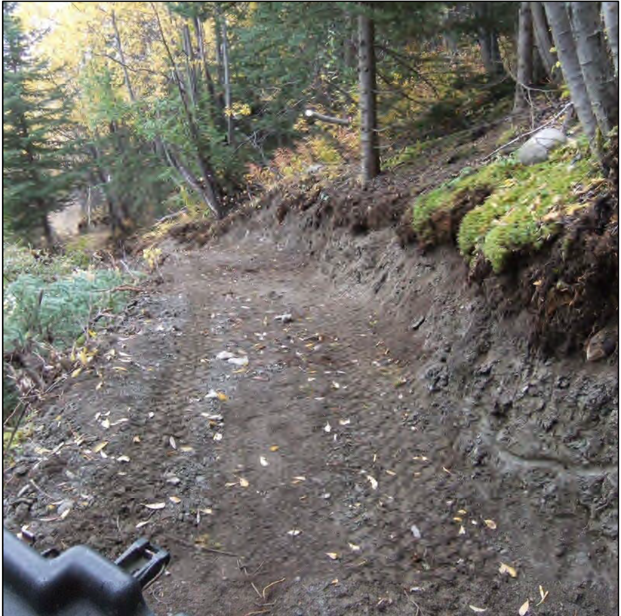
Pic #1, Exploration Trail Construction Between TR 21/15 and TR22/15
