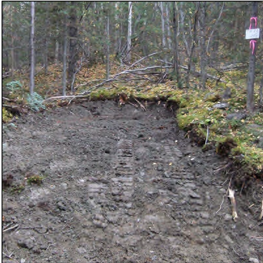
TR22/15, Filled In, Trench Marked with a Pink Ribbon on a tree with a Labelled White Board
