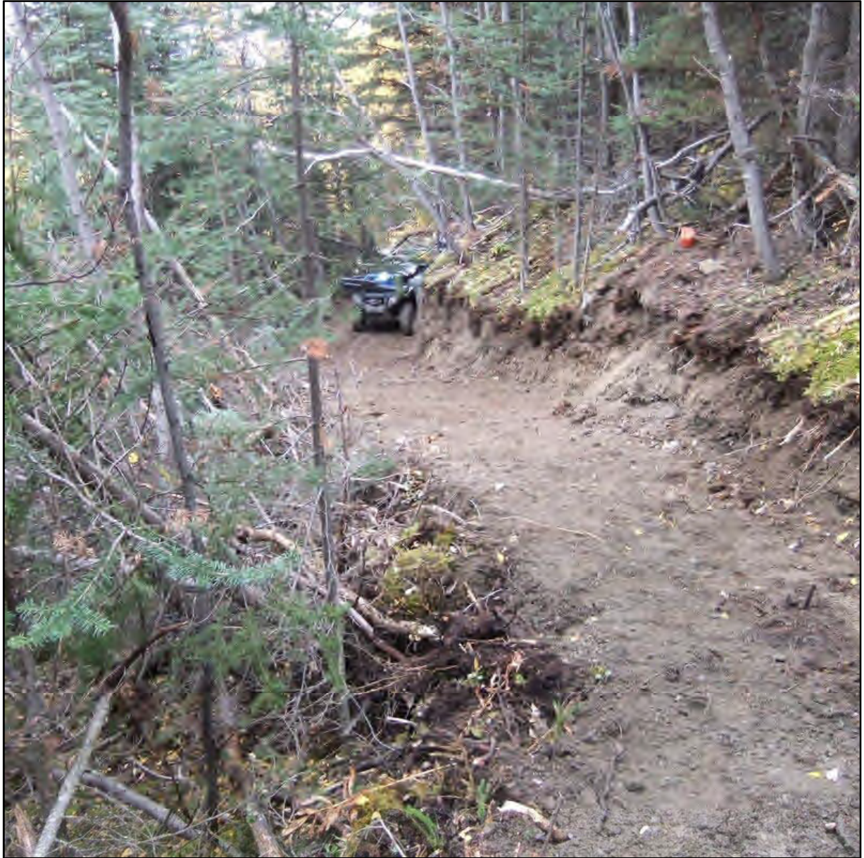
Pic #2, Exploration Trail Construction Between TR 21/15 and TR22/15
