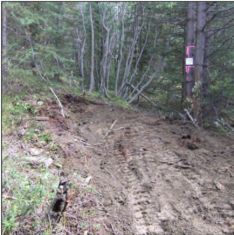
TR18/15, Filled in, Trench Marked with a Pink Ribbon on a tree with a Labelled White Board
