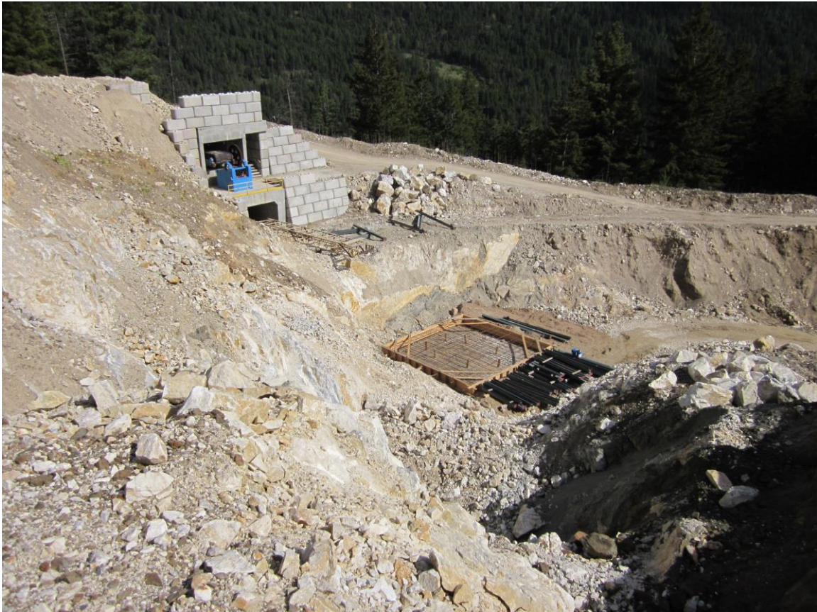
Figure 1. – Photo of Western Canada Limestone Ltd. Crushing Station Under Construction(June 2015)
