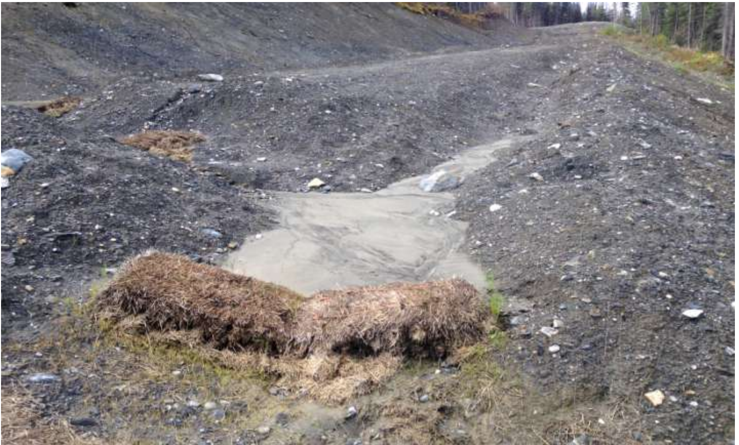
Water Bar and Ditch block (Befor)
