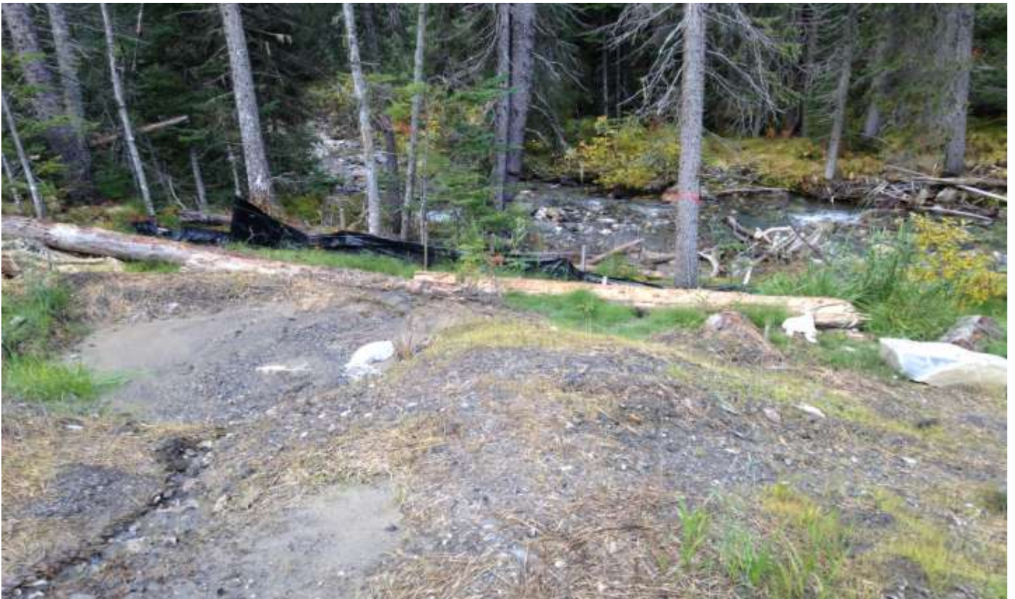
Large Catch Basin above creek (Befor)
