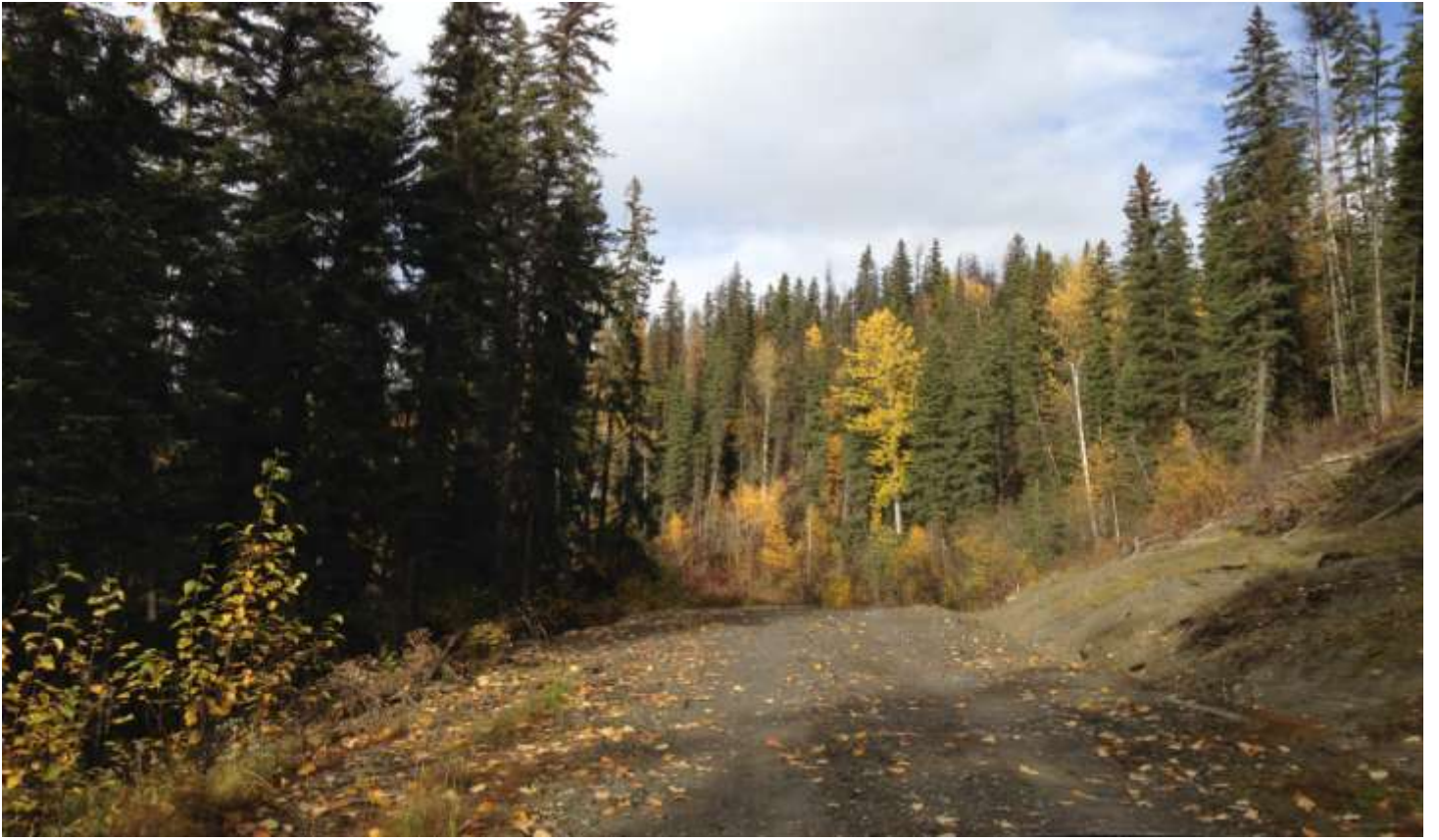
Approx 1.5km on the 4000Rd ( After)
