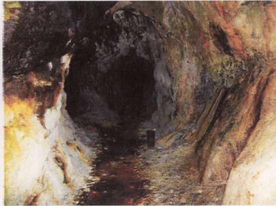
Inside adit, 20 meters
