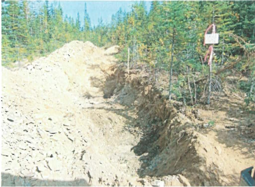
Figure 11 Exploration Trench #TR25/16.
