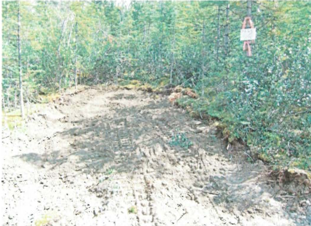
Figure 10 Exploration Trench #TR24/16 Marked and Filled.
