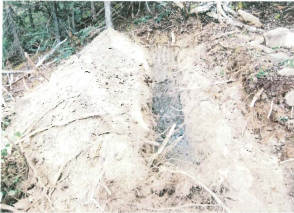
Figure 5 Exploration Trench #TR23/16.
