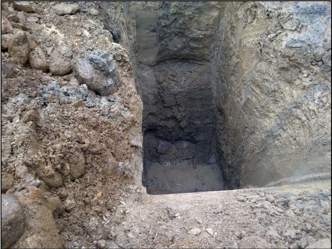
Figure 17 Old Shaft through the Tan Silt and Blue Till to bedrock
