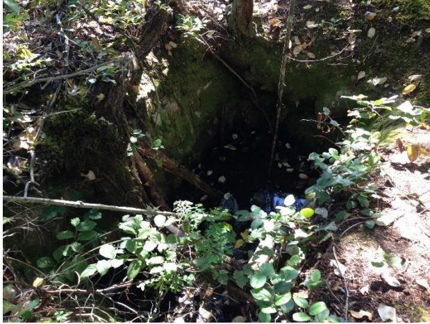
Water filled shaft. Unknown depth. Believed to be a shaft backfilled by Canpac resources.
