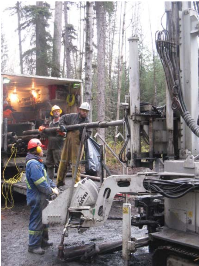
Figure 7: Adding rods to the articulating drill head.
