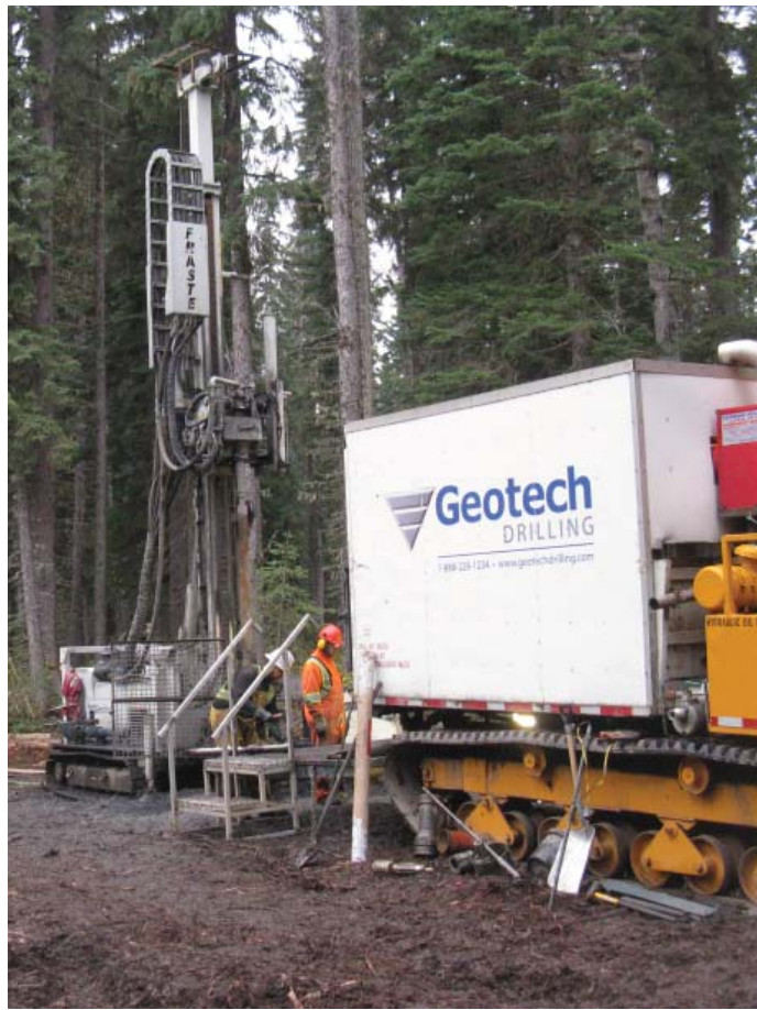
Figure 8: Utility Marooka positioned opposite trackdrill.
