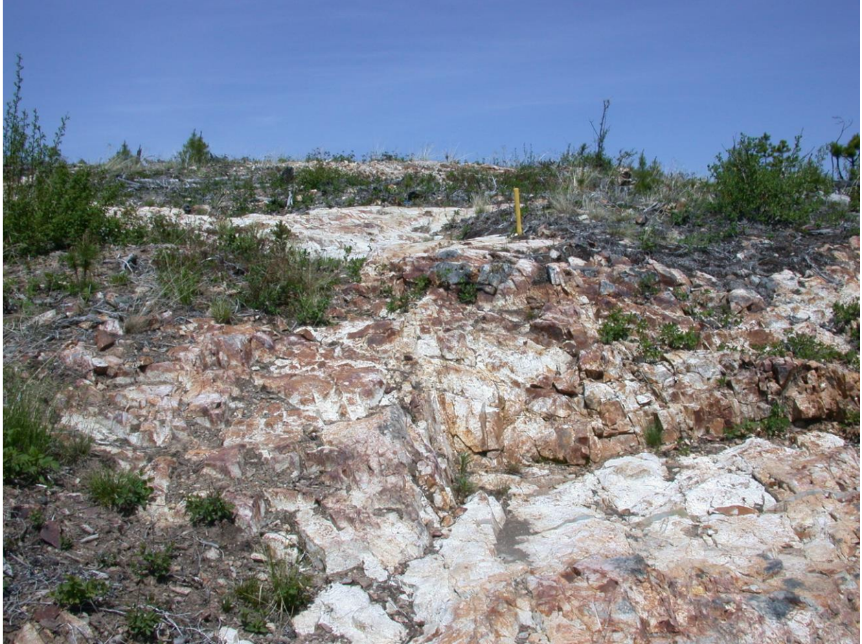
Fox E trench looking 010 azimuth from south end of exposure. Note brittle deformation of host rhyolite and variable limonite alteration.
