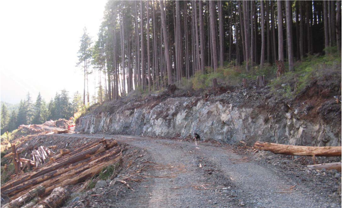
Figure 9: Road cuts in new logging areas within Parson Bay Formation Dark weathering limestones and calcareous crystal tuffs are poorly bedded through much of the section that dips into the foreground.
