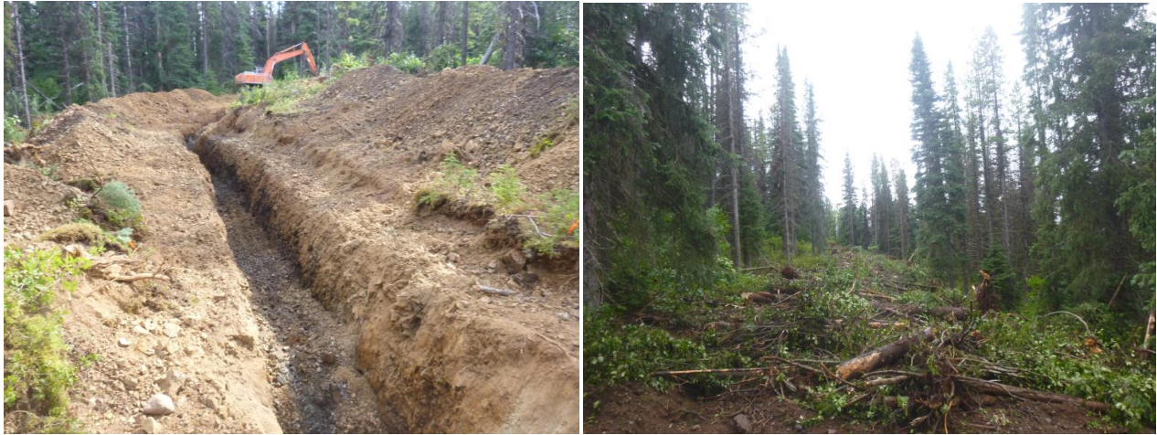
Figure 23. Photographs Trench 4. Left: Trench 4 under construction. Right: Trench 4 reclaimed.
