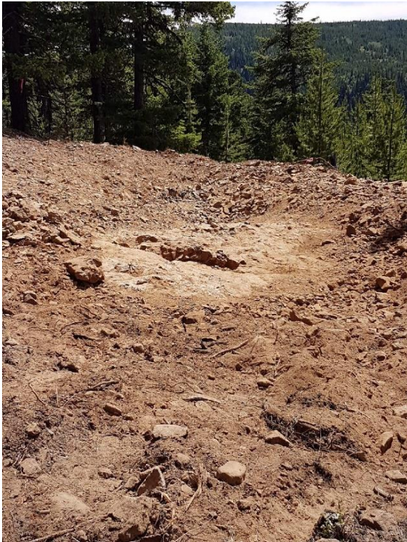
Example of active exploration trench at JR Zone that remains open. Side cast has been contoured.
