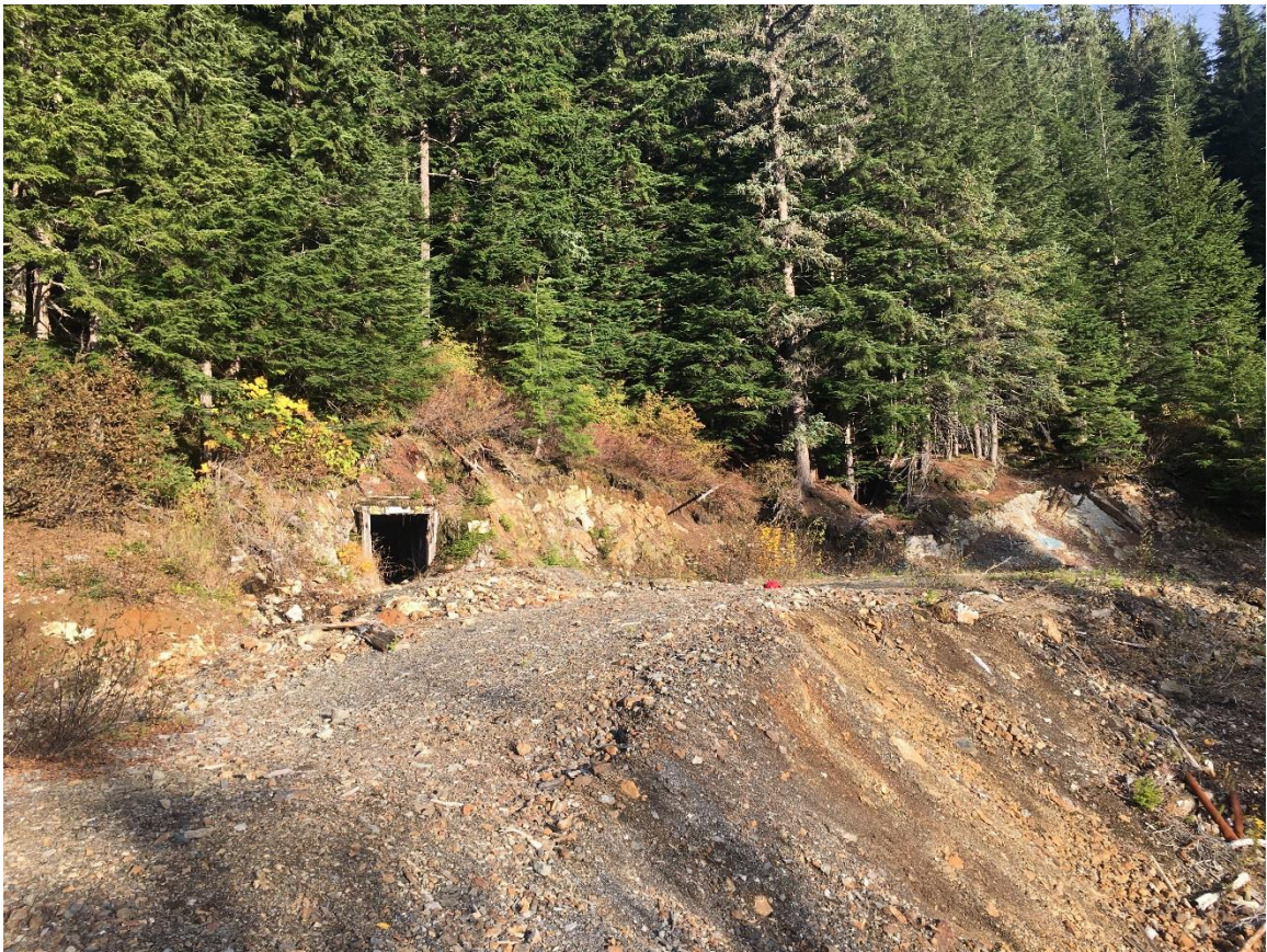
Photo 1: Number 4 (Main) Adit
