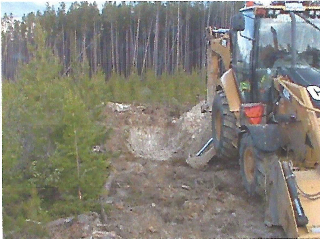
Trenching at the Rome location
