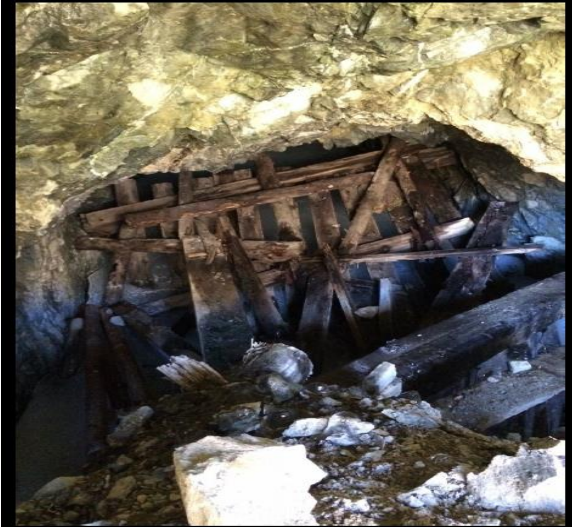
Lowest most adit entrance – boarded up entrance showing signs of collapse
