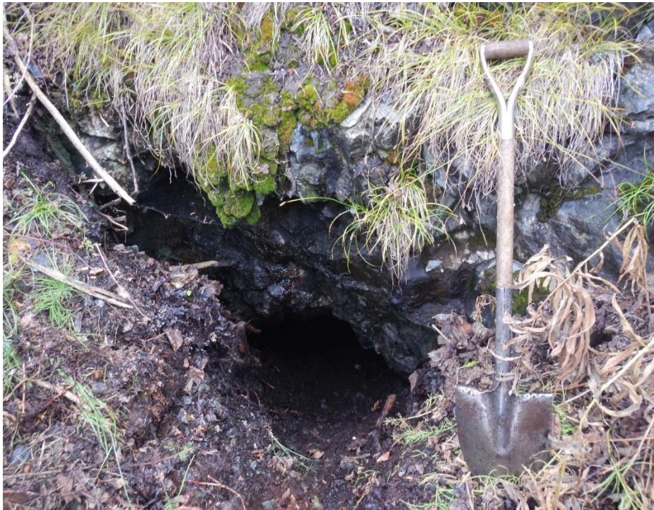
Figure 10: Uncovered French Adit entry
