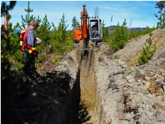
Excavating trench PM1
