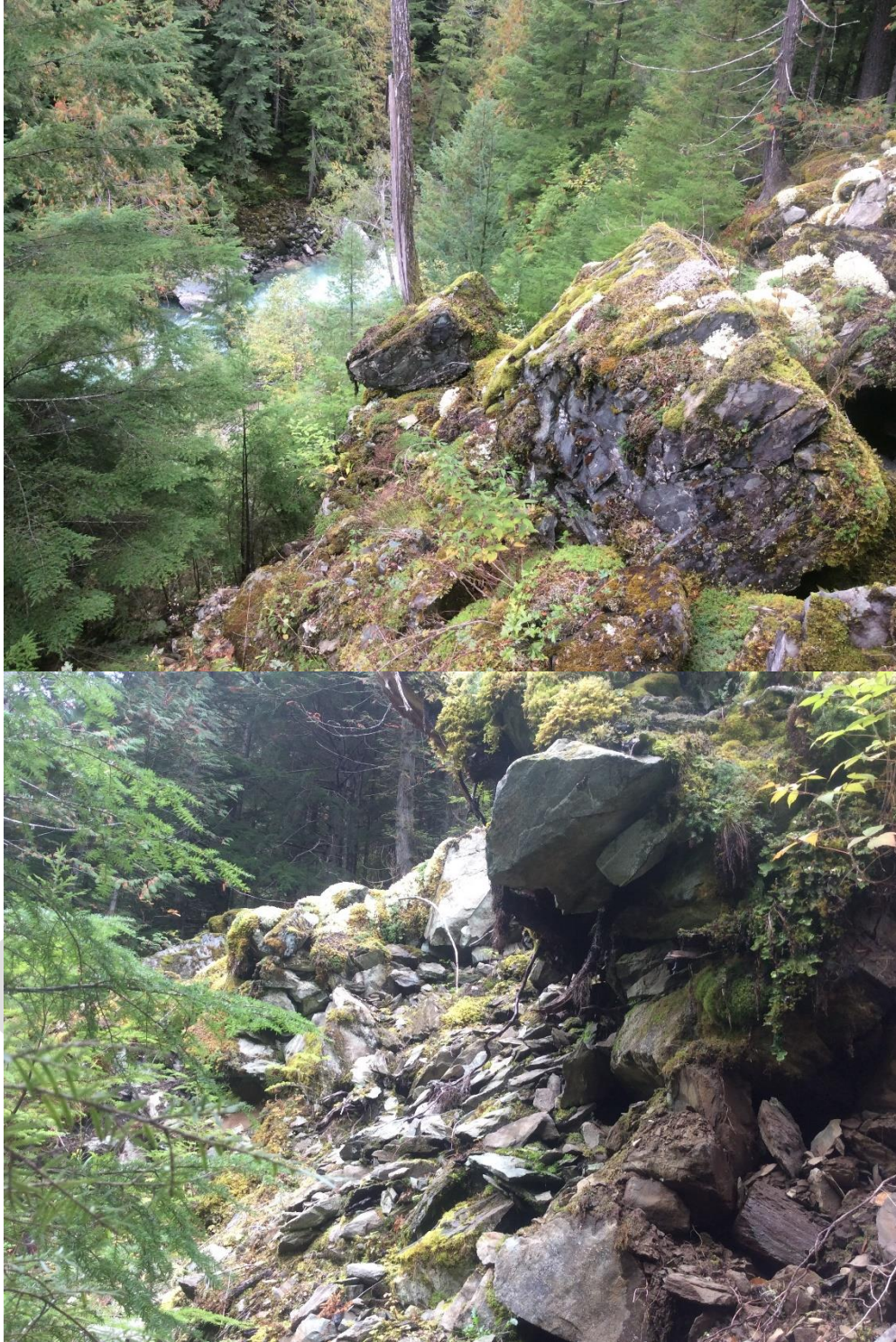
Figure 4: Unstable Rock Fall Debris. Note this is situated approximately 30m above the road. No stopping zone must be extended below this site.
