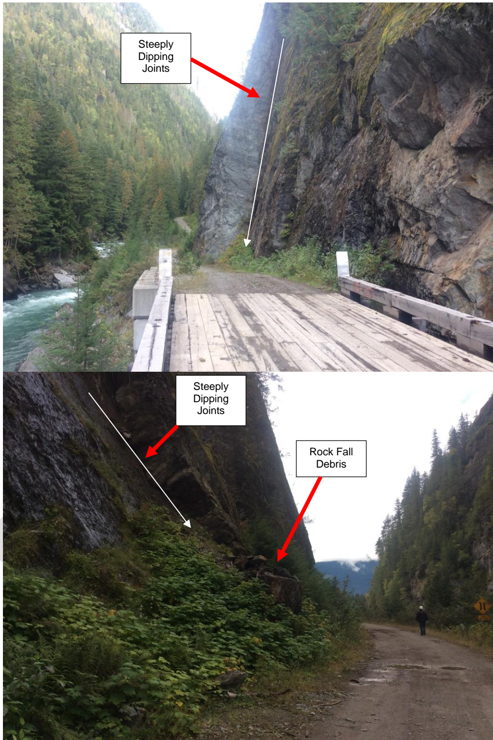
Figure 2: Intrinsically Unstable Rock Masses throughout Canyon Examples. Note steeply dipping joint sets and steep canyon walls.
