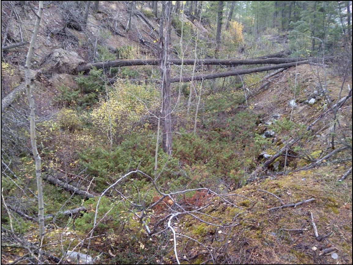
Figure 5 Stone-walled Reservoir near the Southern End of Victoria Ditch probably constructed in 1892, for location adjacent with the Main Hydraulic Pit, see Figure 4
