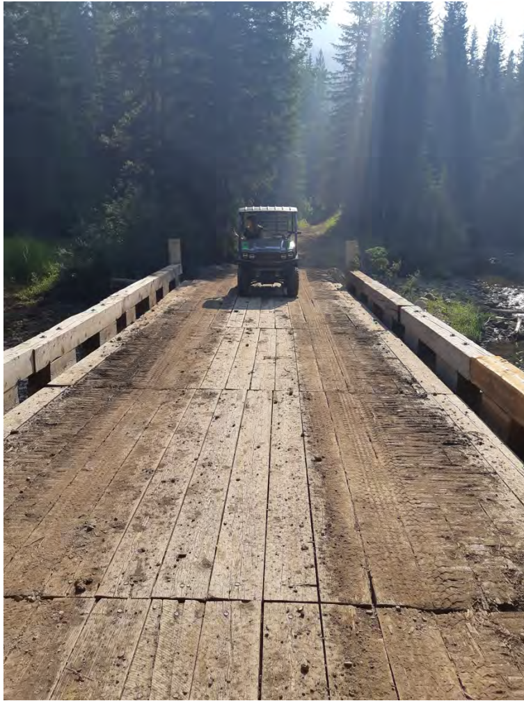
Michel Creek Bridge 2018
