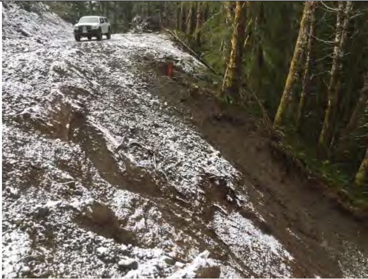
Photo 1 – Slide path blocking further vehicle access
