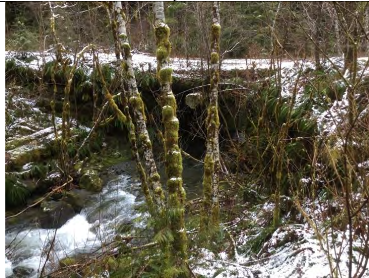
Photo 4 – Seven Mile Creek log stringer bridge.
