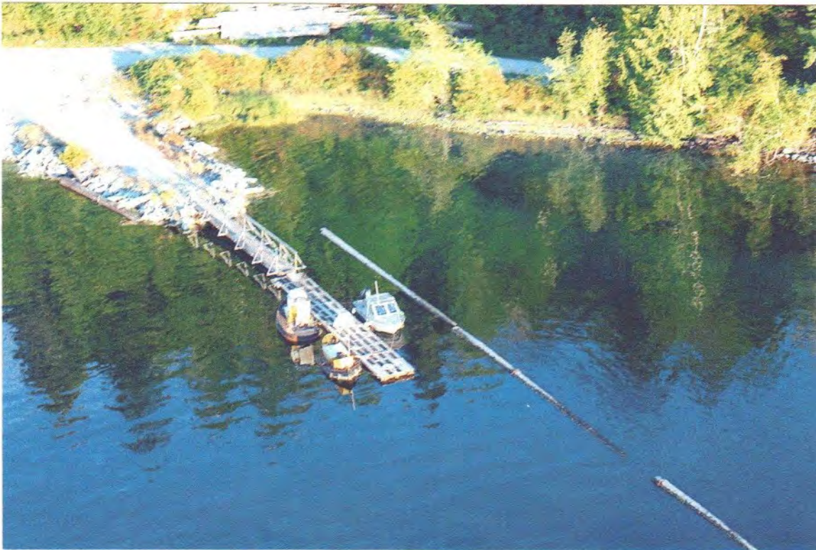
Photo 3: Private Wharf for Logging Operations
