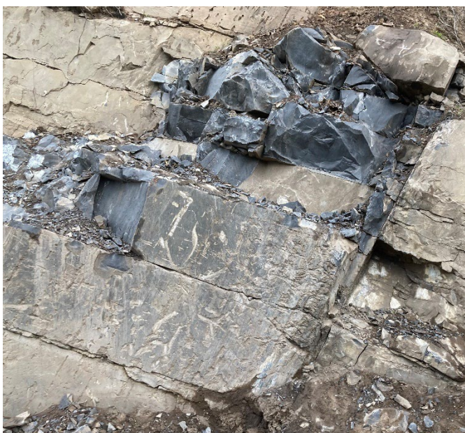
Figure 6 Blocky material near Area 3
